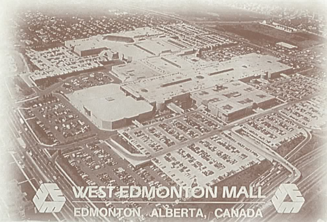
West Edmonton Mall as it appeared with the completion of phase three in 1986.
