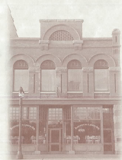
Gainer Block in Old Strathcona was constructed by pioneer industrialist John Gainer in 1902. It was restored as part of the overall renewal of Whyte Avenue between 104th and 103rd Streets.
